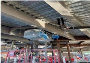
Image 4: Interior duct work hanging ceiling
