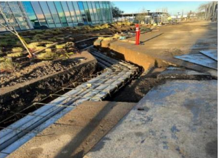
Images Electrical pathway run in front of MS3 installed
