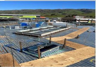
Image 1: Roof top curbs prepped for AHU's
