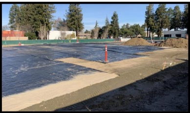
Image 1: Site Work for New Building - Pad Complete and Protected
