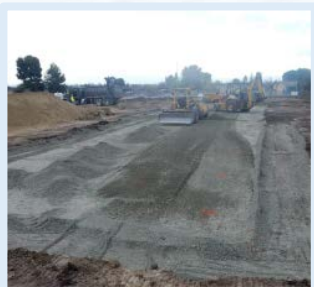
The preparation of the building pads during the week of February 15.
